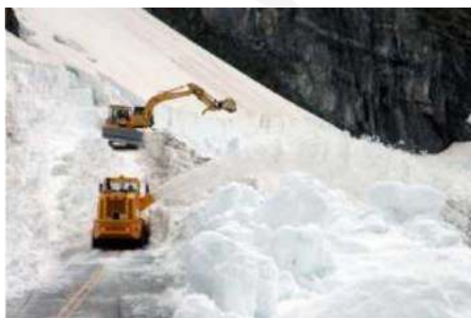
Removing snow from blocked roads. Before manually removing it, salt is spread on the snow cover to ease the job.
